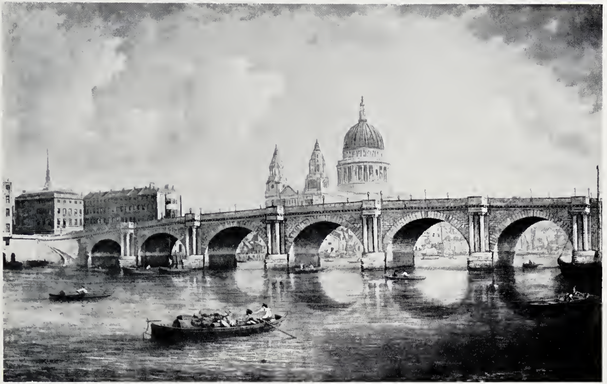
41. MARLOW Blackfriars Bridge
